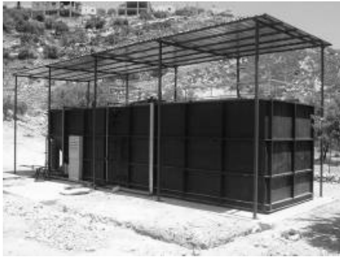
Photo (1): Inauguration of the Wastewater Treatment Plant (WWPT) in Nahhalin village
