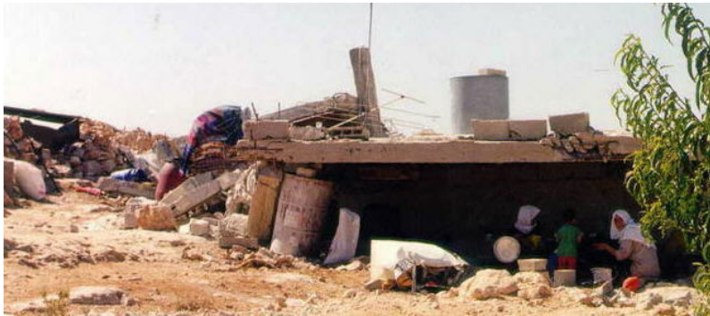
Figure 4: 'Atta's House after demolition.
