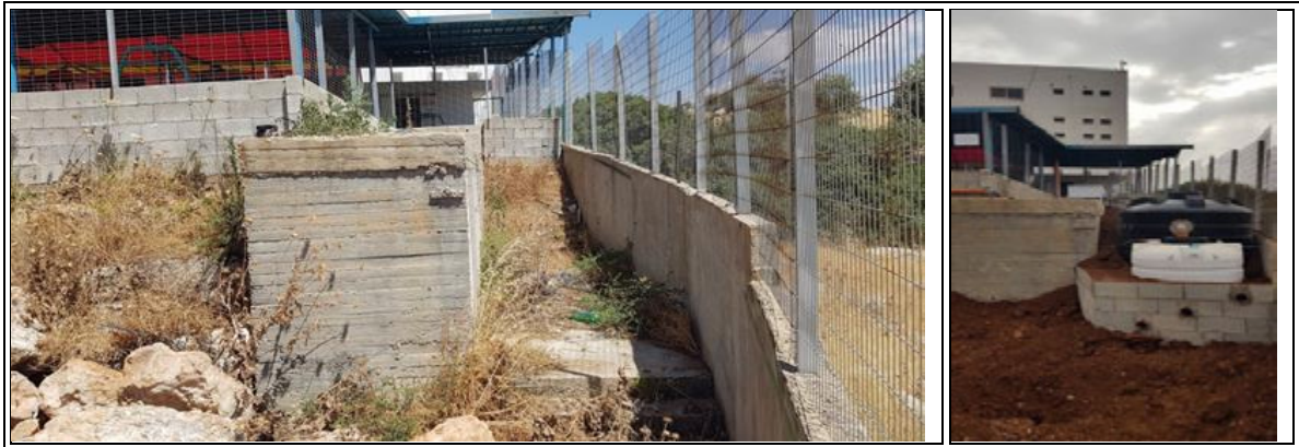
Figure 4: one of the three implemented wastewater treatment plants through The Arab Fund Project – Location : Al- Aqaba Tubas Governorate (after and before) .
